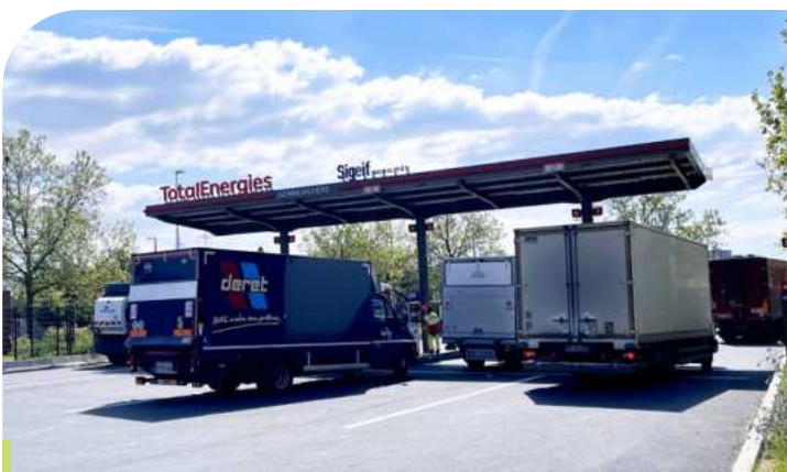
Station GNV-Bio-GNV à Gennevilliers.
